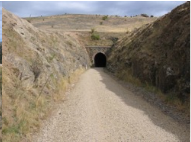
Entrance of 1 st Poolburn Tunnel
